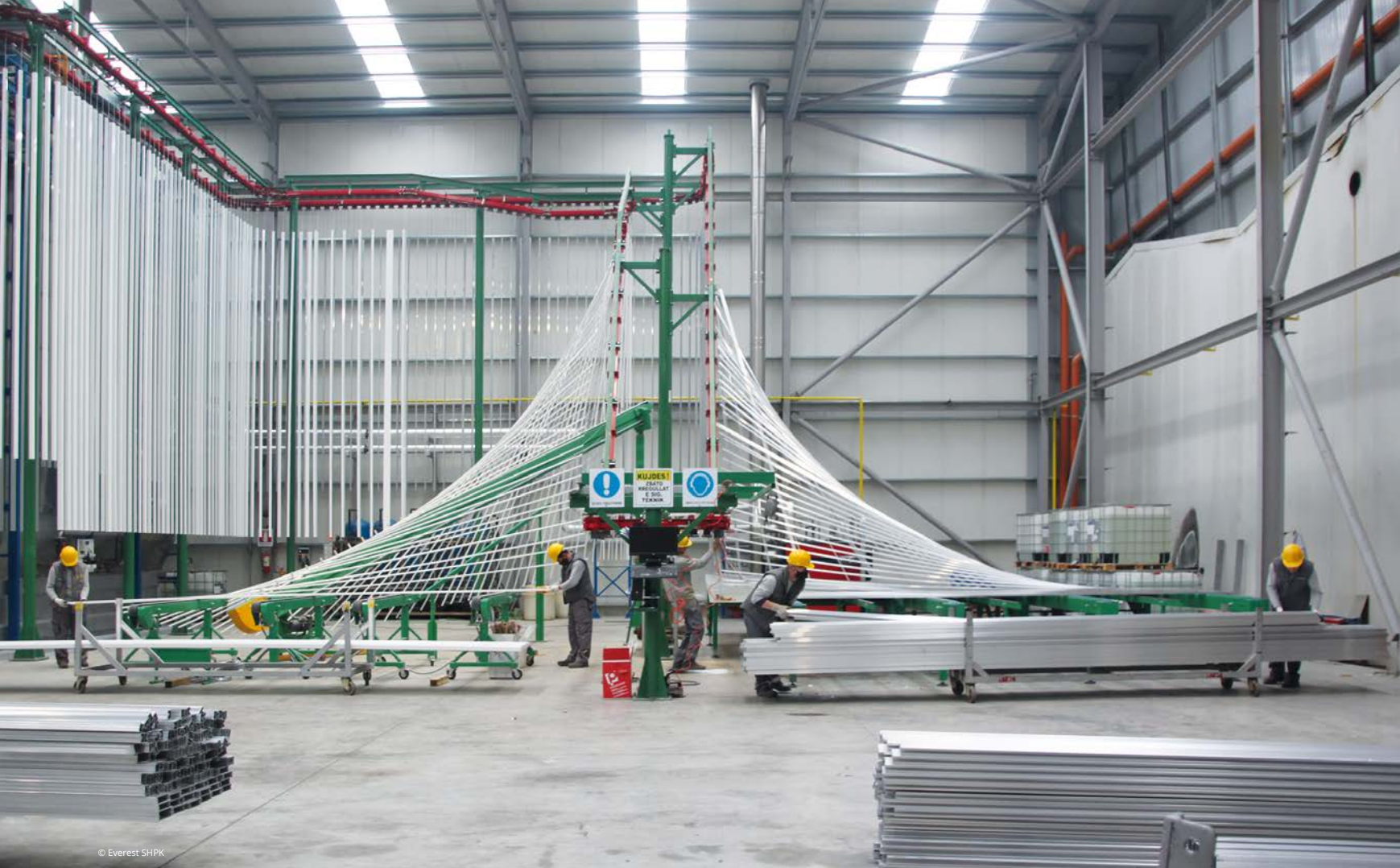
Loading and unloading area of the SAT vertical coating system for aluminium profiles manufactured by Everest.
