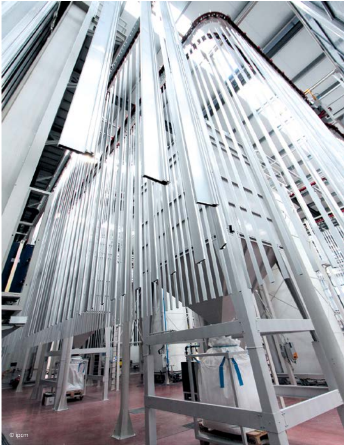
Profiles exiting the pre-treatment tunnel.
